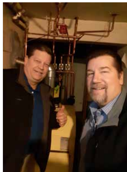
Charley Holmes (left) and Tom Raulinavich showing off the new boiler
